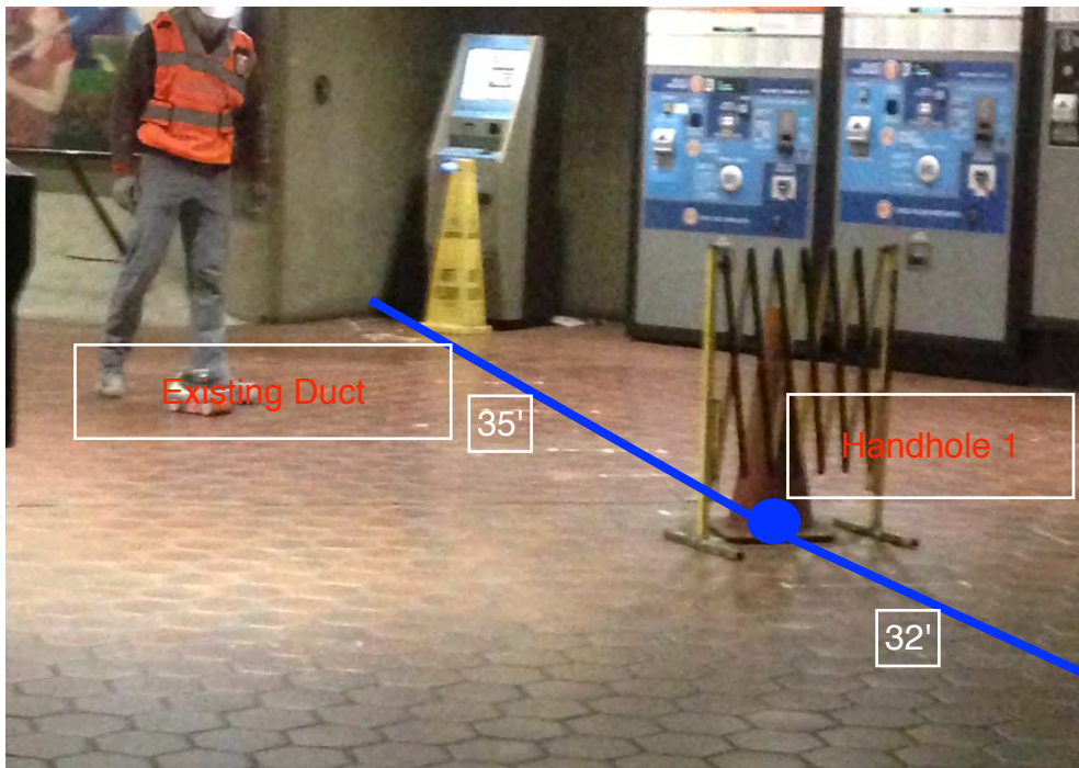
Photo #2 – Existing duct run on mezzanine floor
